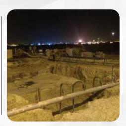
WellPoint systems are a commonly used dewatering method as they are applicable to a wide range of excavations and groundwater conditions
