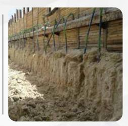
The main components of this type of shoring system are vertical steel wide flange beams known as soldier piles and horizontal timber lagging. The soldier piles can either be placed in drilled holes or installed by driving the beams in the ground. The soil must have sufficient cohesion and stability to retain a vertical face until the lagging can be installed between the soldier piles
