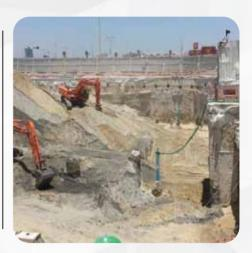
A deep well system consists of an array of bored wells, each fitted with a multi-stage electric submersible borehole pump. As water is pumped from each well, the groundwater is lowered creating a cone of depression or drawdown around itself.
