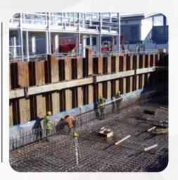
Sheet piling is a form of driven piling using thin interlocking sheets of steel to obtain a continuous barrier in the ground where is the soil condition poor.
